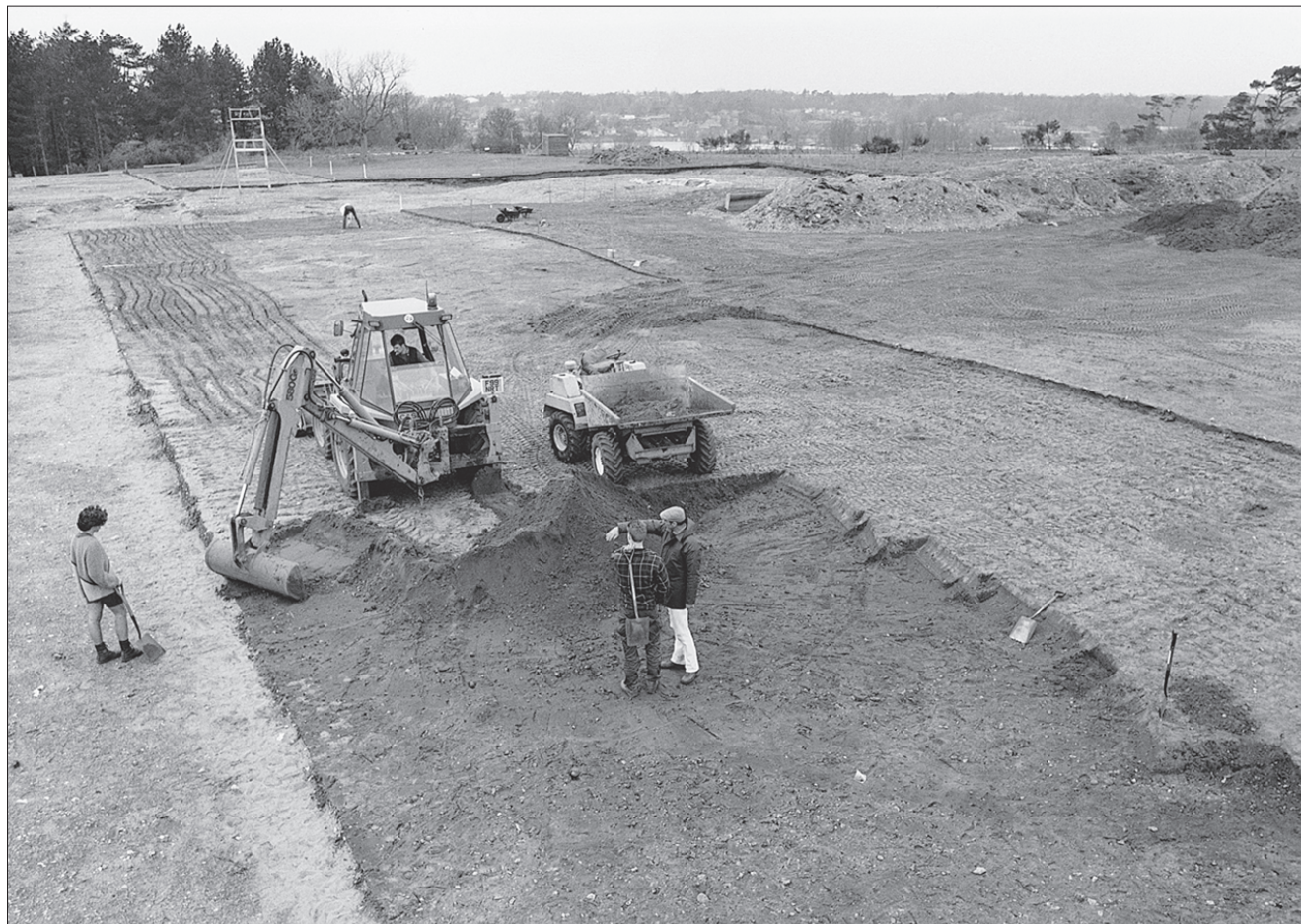
Plate 11 Opening the site by machine: (a) a back-hoe served by a dumper, used to remove ploughsoil on Int. 39; (b) use of a machine in the scheduled area (Int. 48), following the confirmation that the turf covered an old ploughsoil. The tracked excavator, a 'Drott', right, removed the turf and then 'ploughed' the surface with the fork on its front bucket. The surface was systematically fieldwalked (background) and metal-detected, and then removed by back-blading (right). On the left, a trowelling-line prepares Horizon 2 on Mound 6.
